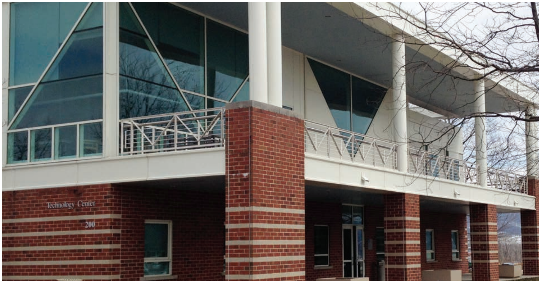
The Technology Center in Innovation Park
